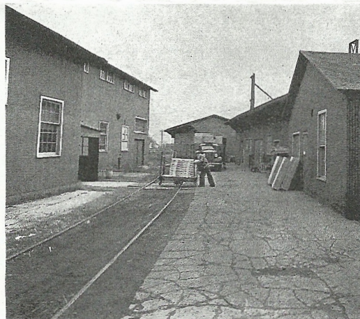
The Uline factory consists of ten little red buildings strung along the railroad tracks, with a single siding. Mr. Uline made $55,000 in 1928, lost money every year during Depression, hopes to make about $2,500 this year.
