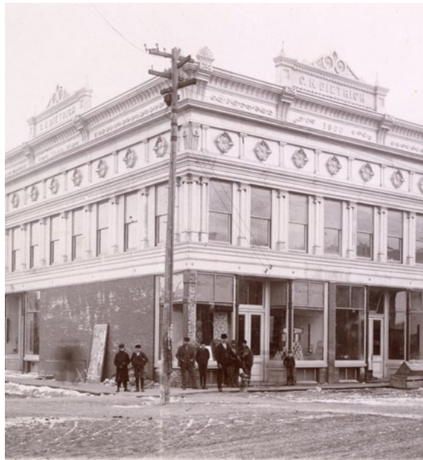
Historic Dietrich building
