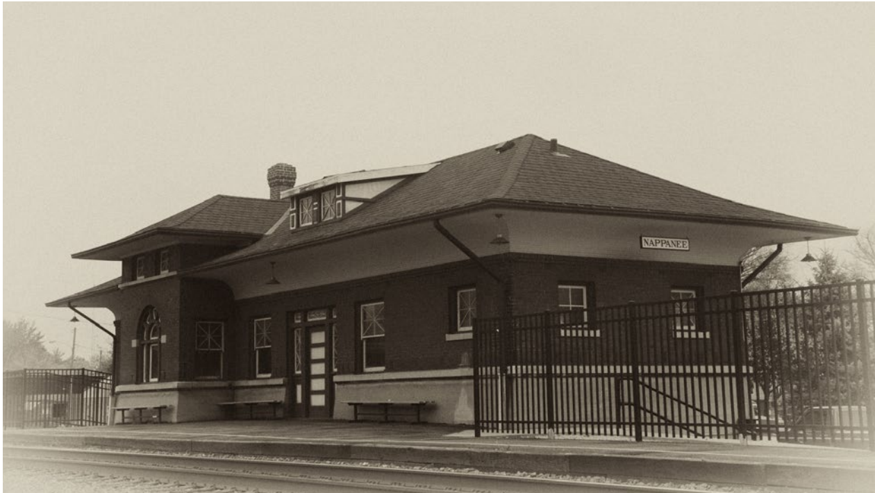
B. & O. Railroad Depot, 1910
