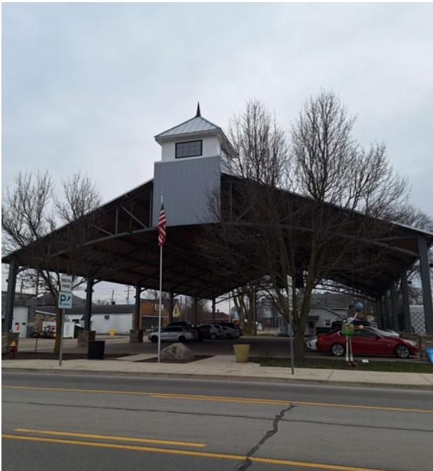
Existing downtown pavilion, Nappanee, IN
